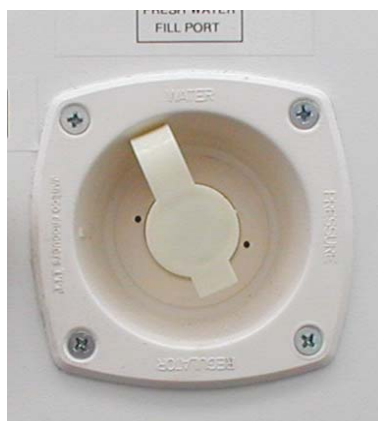
Figure 51: Humidifier External Water Connection
