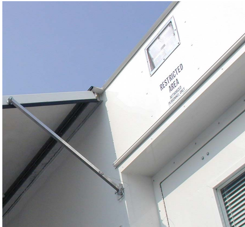
Figure 64: Staff Door Lighting
