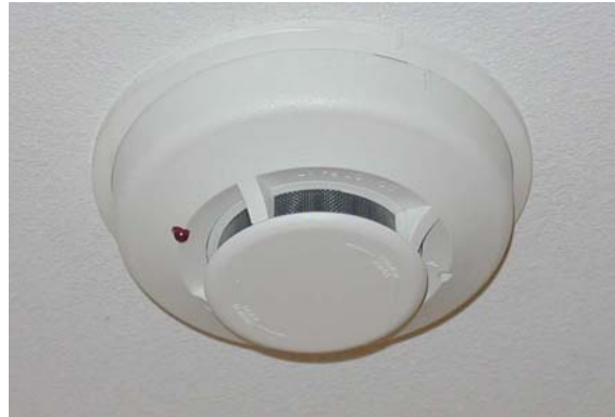
Figure 31: Smoke Detector
