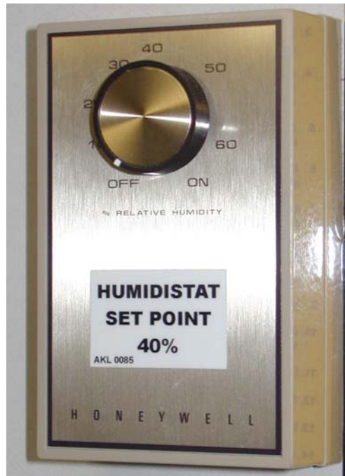
Figure 52: Humidity Controller
