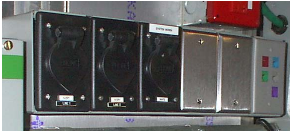
Figure 25: Phone and Data Line Connections (Typical)
