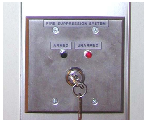
Figure 36: Maintenance Switch
