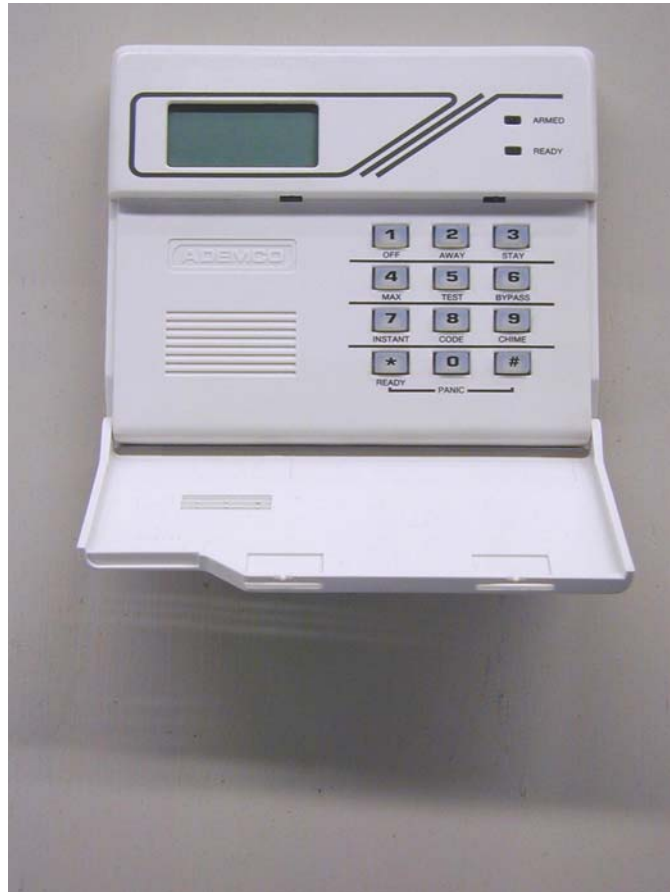
Figure 39: Intrusion Alarm Keypad
