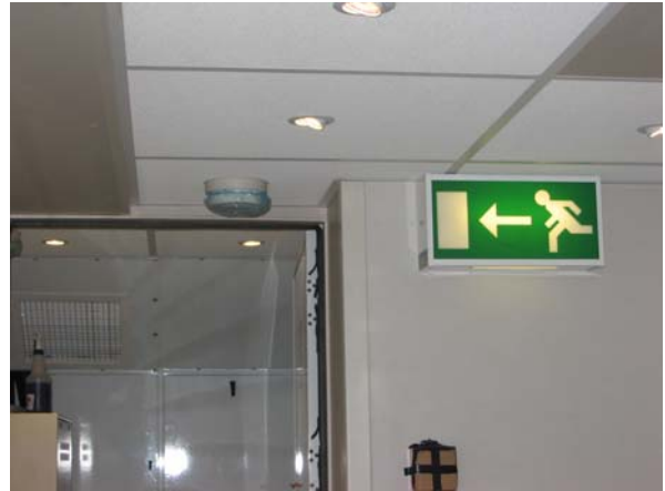
Figure 47: Control Room Lighting
