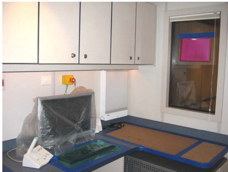
Figure 12: Control Room Overall
