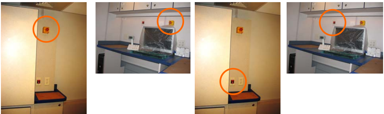
Scan Room and Control Room Guarded Magnet Quench Buttons
