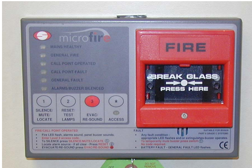
Figure 6: Fire Alarm Control Panel
