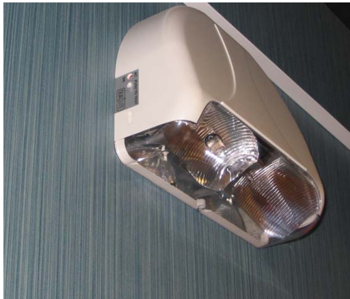
Figure 2: Emergency Lighting (Typical)
